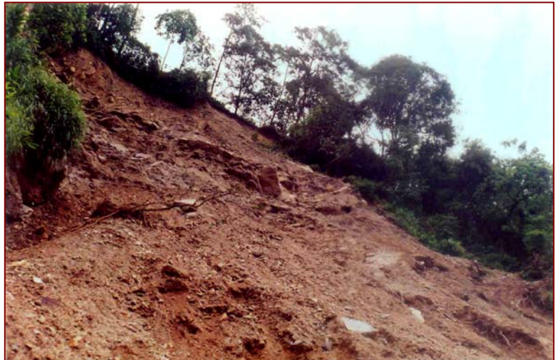
Photo: Slope failure due to heavy surface runoff
