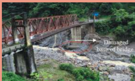
Damage of under Construction bridge at 14 th mile of the watershed
