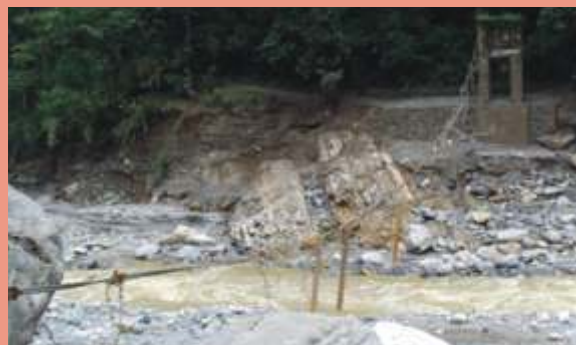
Destruction of Suspension bridge connecting Namrung village to Palung village
